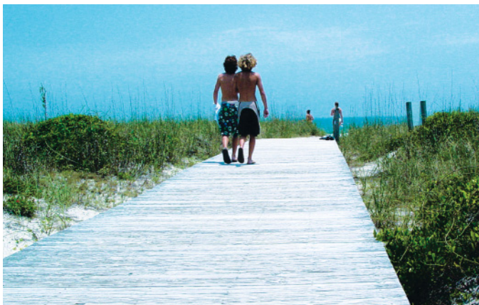
Photo 18: This is an on-grade walkway without railings.
